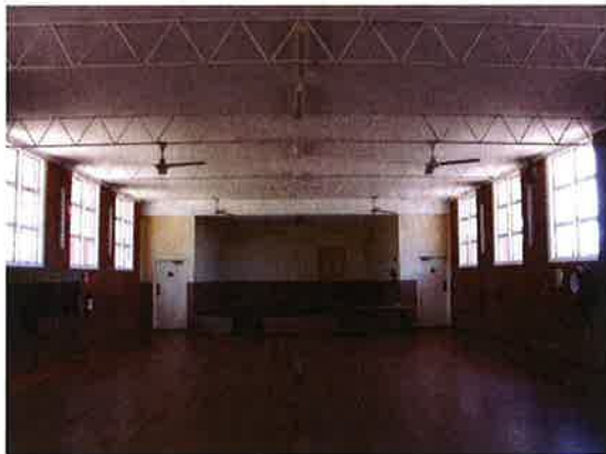
Figure 5.132 Interior of the hall, with stage at the far end.
