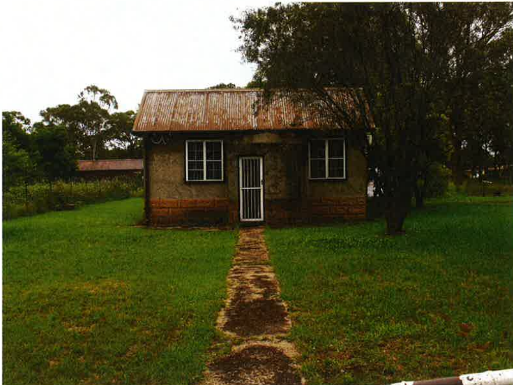
Figure 5.157 The cement rendered house at 40 Browns Road.
