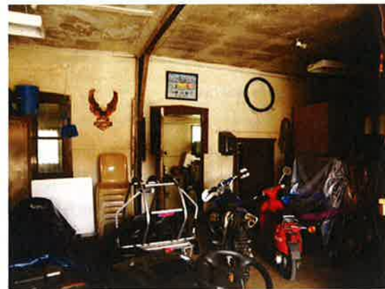
Figure 5.199 Interior of the rear building, now used for storing vehicles. Note original architraves around doors and windows.
