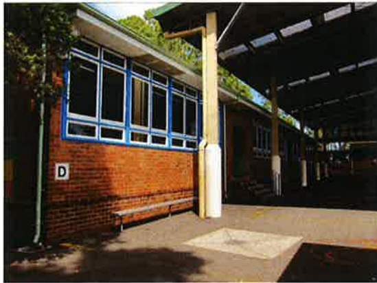
Figure 5.115 Building D, Classrooms, north side.
