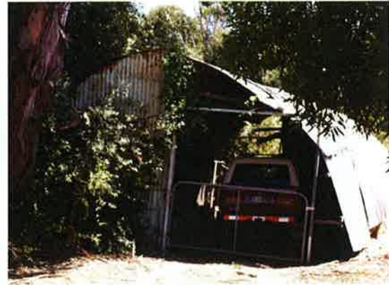
Figure 5.173 Nissen hut on Bringelly Road; the east end has been modified to provide parking access.
