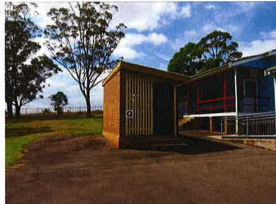
Figure 5.114 Ablution shed (Building Q).
