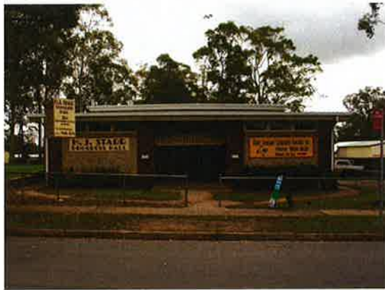
Figure 5.128 View from the street.
