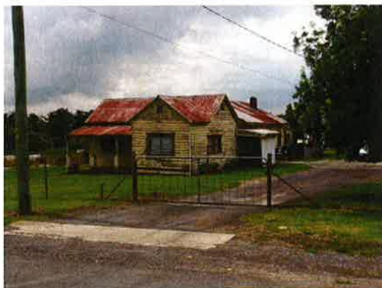
Figure 5.198 View from the southeast.
