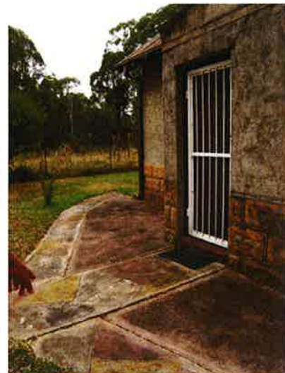
Figure 5.159 Detail of the painted crazy paving path at the front of the house.
