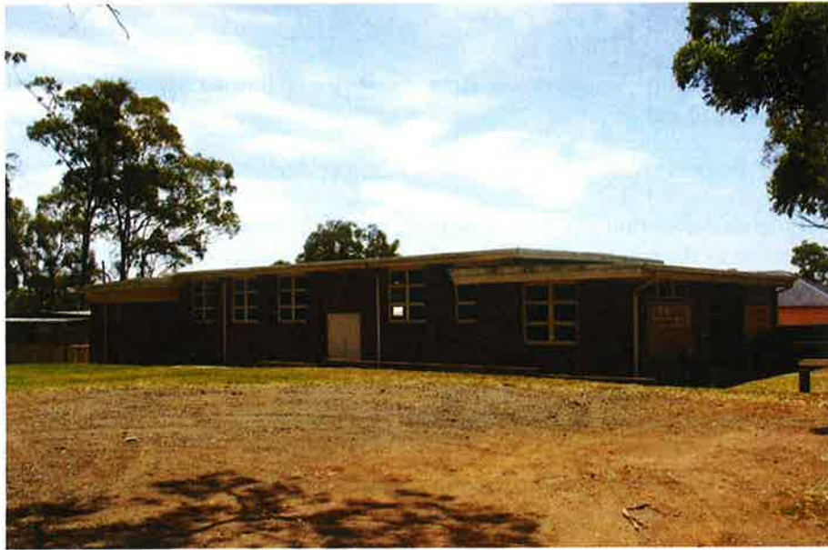
Figure 5.127 H J Starr Progress Hall, view from the southeast.
