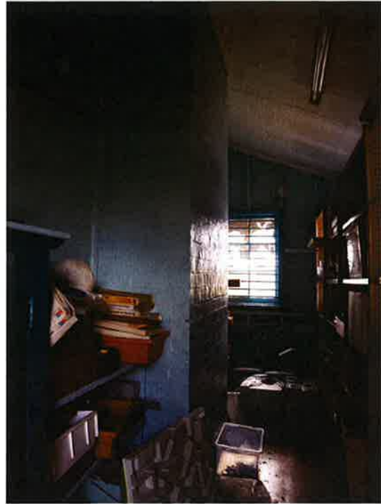
Figure 5.106 Interior partition and rear of brick chimney.
