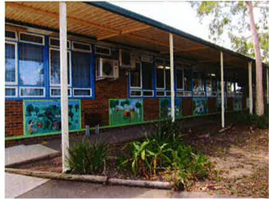
Figure 5.116 Building D, south side.
