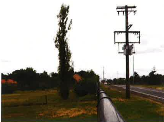
Figure 5.192 View to the house along Fifteenth Avenue to the east.
